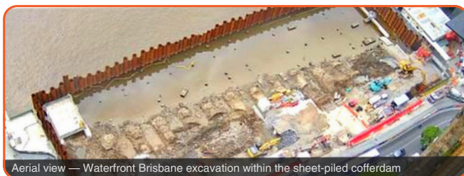
Aerial view — Waterfront Brisbane excavation within the sheet-piled cofferdam
