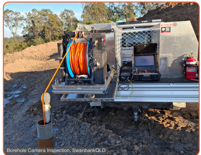
Borehole Camera Inspection, SwanbankQLD
