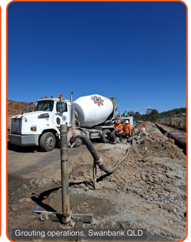
Grouting operations, Swanbank QLD
