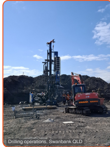
Drilling operations, Swanbank QLD
