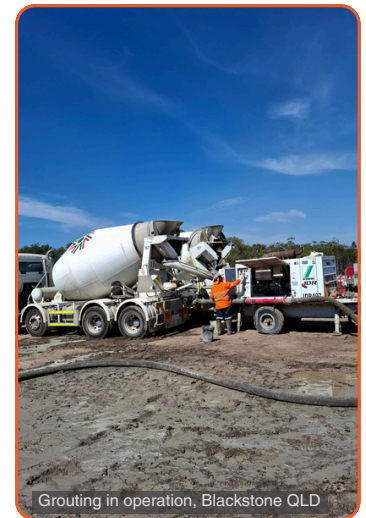
Grouting in operation, Blackstone QLD
