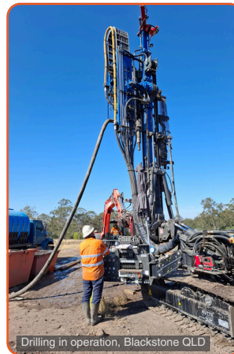
Drilling in operation, Blackstone QLD
