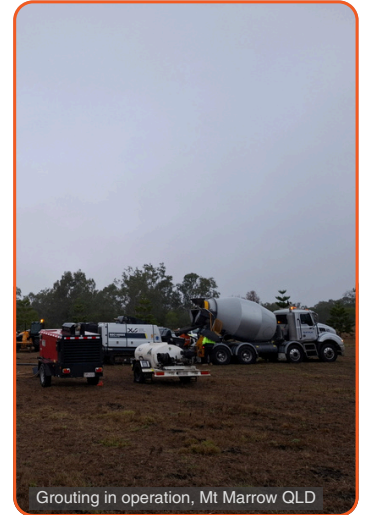
Grouting in operation, Mt Marrow QLD
